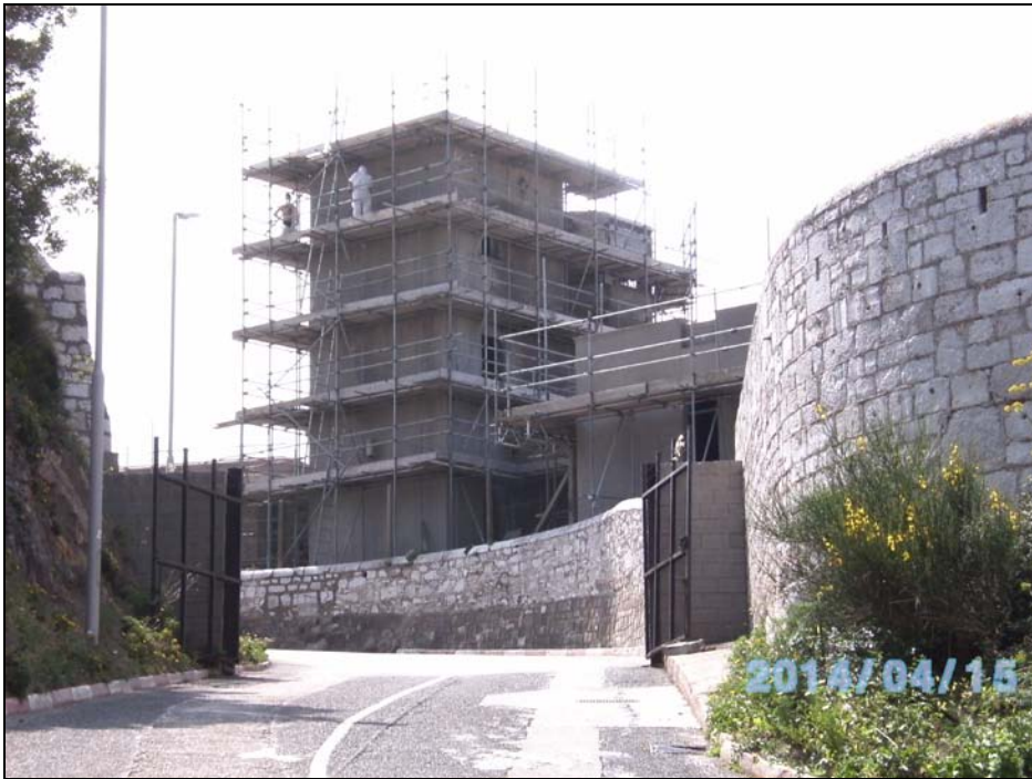
Plate C-03 – Looking south from Windmill Hill Road.
