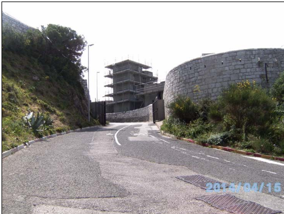
Plate C-02 – Looking south from Windmill Hill Road.
